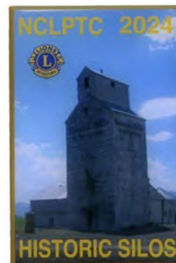
FG 1201 24 Bob Walker (SC) Silo # 7
